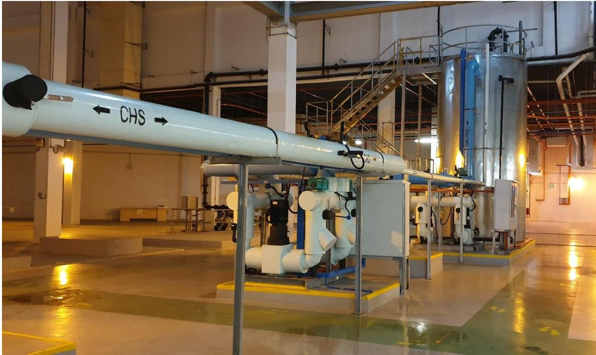
*The Phase-Change Material thermal energy storage system installed at Keppel DHCS' Changi Business Park District Cooling Systems plant.
