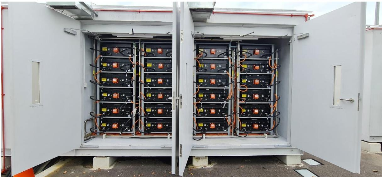
*Battery Modules within the Battery Container*
