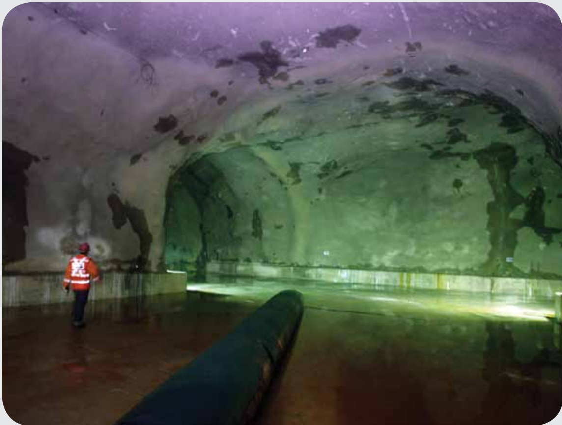
Fig 2.3 Jurong Rock Cavern start-up gallery
