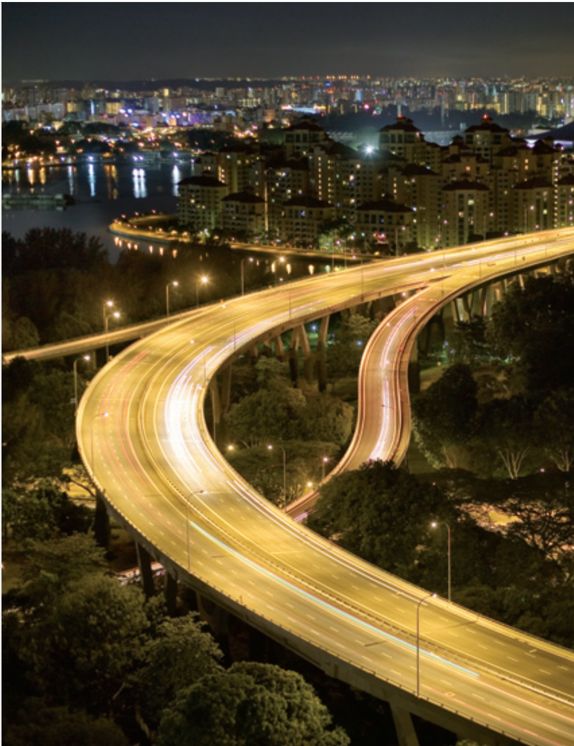
Reliable power supply: up there in world ranking.
