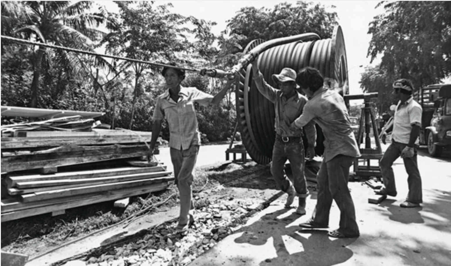
Where would we be without daily-rated workers toiling to lay cables and pipes?
