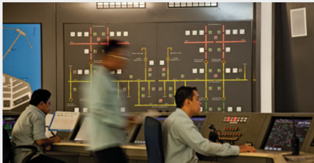
Keeping the electrical system humming along with little margin of error.
